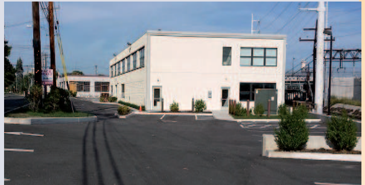
Elinco Corporate Headquarters and adjoining facility in background, all in front of the Fairfield Metro Train Station in Fairfield, CT
